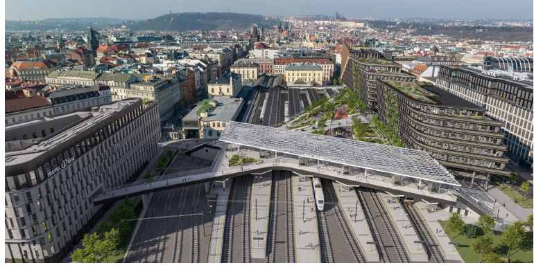
Figure 8 Key project Z1 – Roof over the tracks at Masaryk Railway Station, source: Seznam zprávy, 20. 12. 2023
